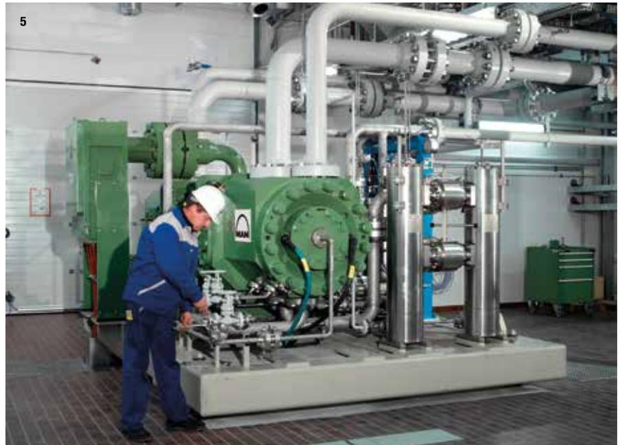
**5** The tandem HOFIM™ offers the added capability of operating the two casings either in the series or in the parallel mode. This allows the operator to cover the widest possible duty range at high efficiencies. Switching from one mode to the other can be effected during operation without shutdown.
