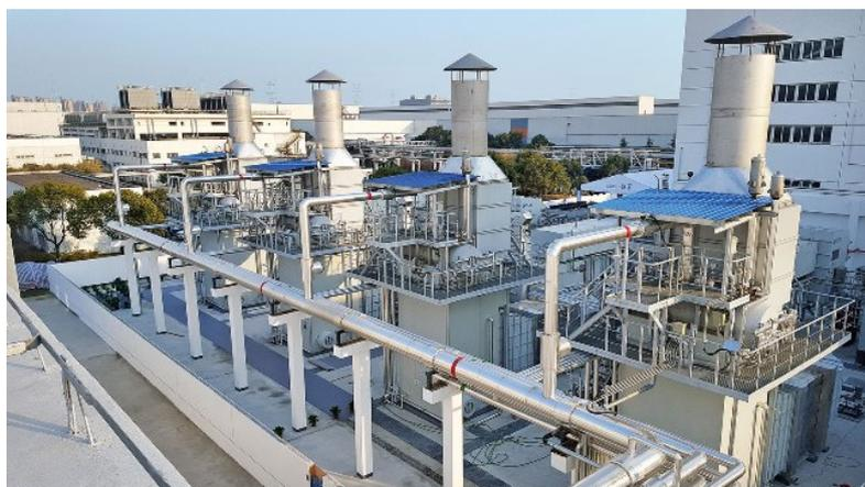
(MAN\_MGT\_VW\_Shanghai.jpg) Four MGT turbines supply electricity and heat to the Volkswagen plant near Shanghai.
