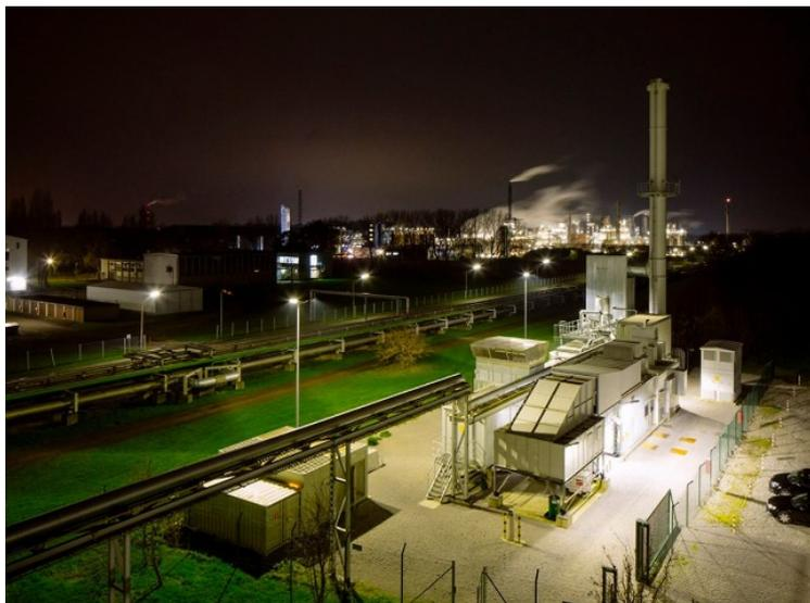
(MAN\_MGT\_1.jpg) As shown at this plant in Rheinberg (Germany), MGT turbines supply electricity and heat in the highly efficient CHP operation.
